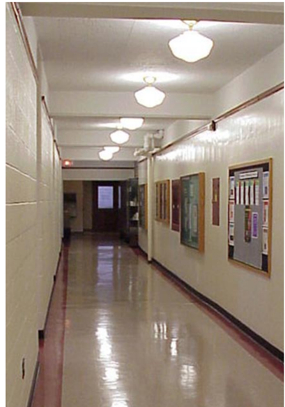
New lights brighten hallway outside rooms 241-245 in Altgeld Hall.
